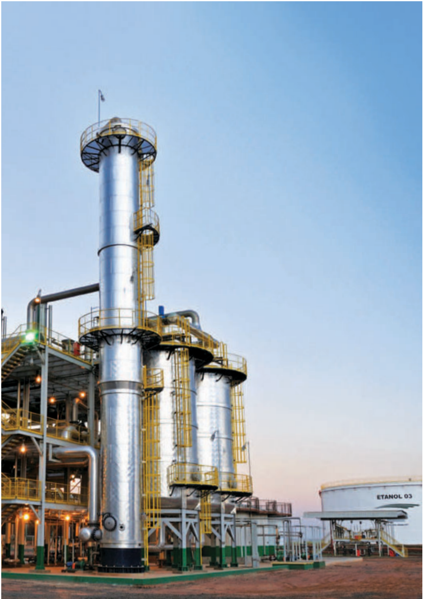
CMAA sugar mill and ethanol plant in Brazil
