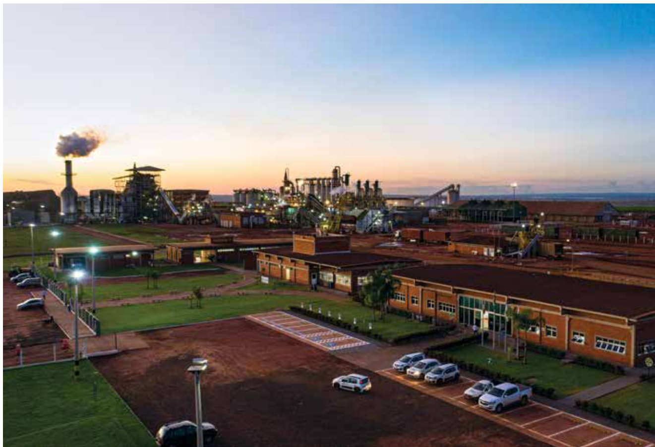
CMAA's UVP sugar mill and ethanol plant in Brazil
